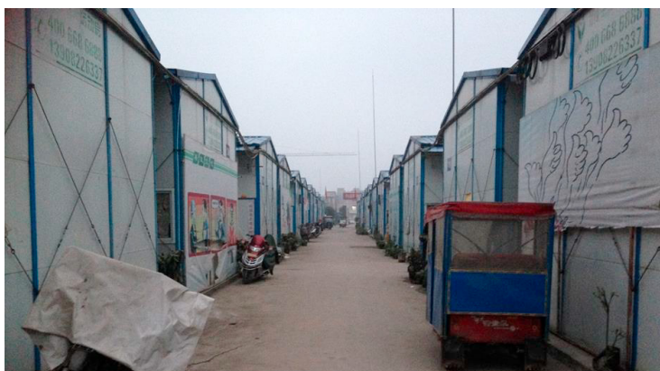
Fig. 1. Prefabricated temporary houses intensively used in disaster relief in the 2008 Wenchuan earthquake in China
