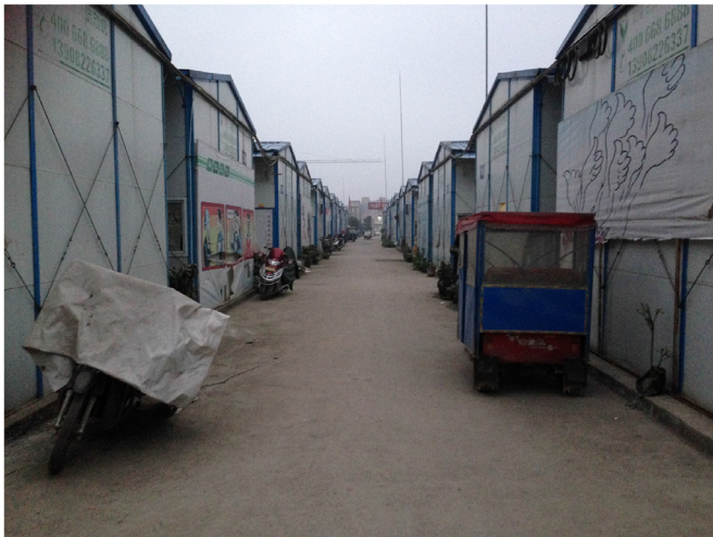
Fig. 1. Prefabricated temporary houses intensively used in disaster relief in the 2008 Wenchuan earthquake in China.
